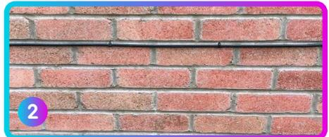
There can be no more than five bends, each at a minimum bending radius of 120mm (the typical radius of a dinner plate) i.e. DO NOT create any 90-degree bends as this exceeds the angle that the fibre cable, that we need to later pass through the conduit, can tolerate.
